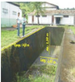
$$\begin{aligned}\text{Vol. Do retângulo:} \\ \text{h} \times \text{c} \times \text{L} &= \\ 2,20 \times 14 \times 2,45 &= \\ 75,46 \text{ M}^3 \\ (\text{Aprox.} &= 76 \text{ M}^3) \\ 76:2 &= 38 \text{ Kg}\end{aligned}$$
